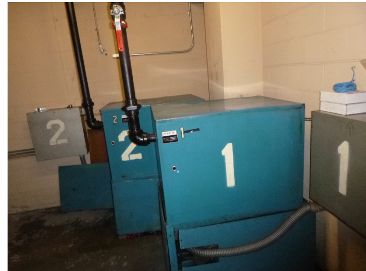
View of the two hydraulic elevator packages.
