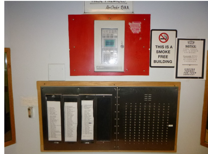
The EST fire alarm control annunciator panel (top) and intercom panel (bottom) located in the entrance vestibule.
