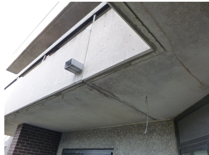
No significant cracking/deterioration was observed at the underside of balconies from available vantage points.
