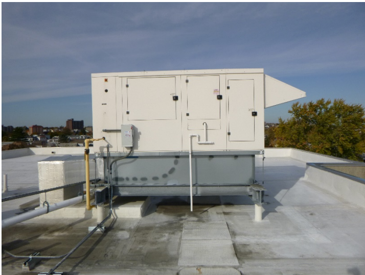
One of three recently replaced Reznor roof mounted makeup air units (MAUs).
