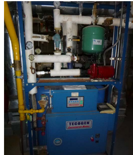
The Tecogen cogeneration system that produces domestic hot water and supplemental electricity for the building.
