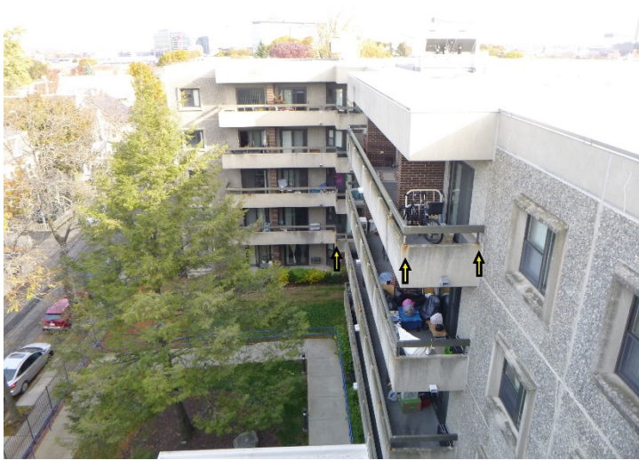
View of the concrete balconies. Concrete surfaces exhibit staining and organic growth. Yellow arrows indicate rust staining near balcony railing mounting brackets.
