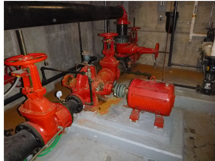
The original 50-horsepower split case fire pump.
