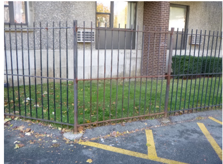
The painted metal picket fencing exhibits age related wear and surface rust.
