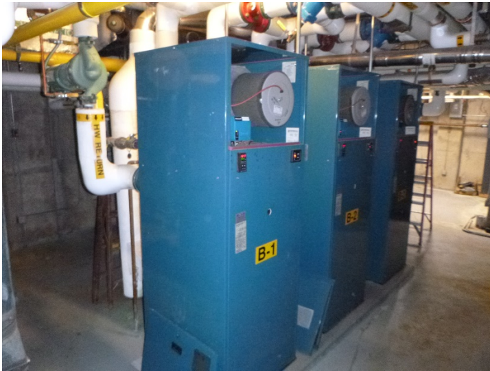
Three Thermal Solution Evolution, modulating, gas-fired boilers produce hydronic heat for the building. Each boiler has a rated input capacity of 1,500-MBH.
