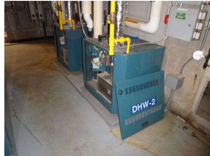
The domestic hot water backup boilers are gas-fired 190-MBH Burnham boilers.
