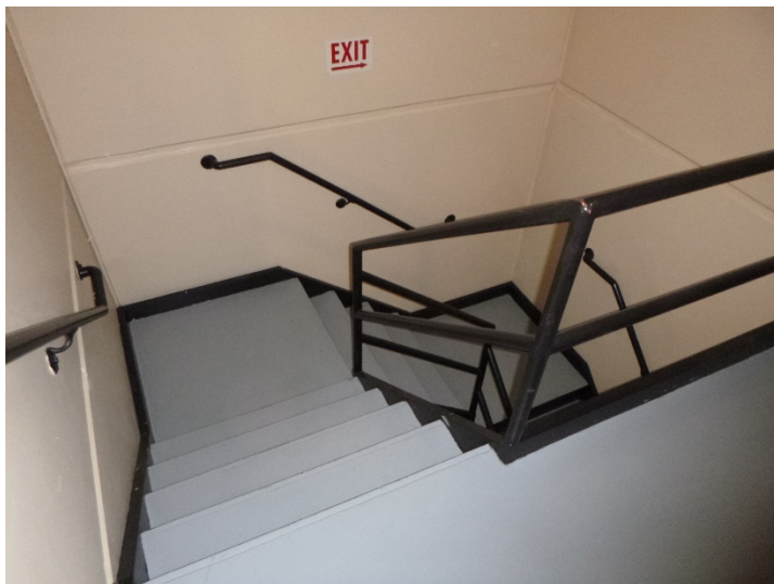
Typical egress stairwell finishes and condition. Note: stairwell railings do not meet current accessibility or safety standards.
