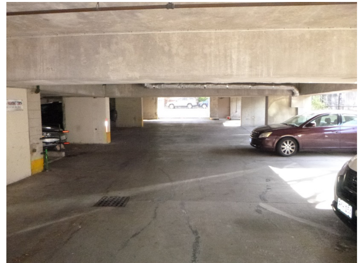
View of the parking garage located under a portion of the building. Note: faded striping and evidence of past repair efforts.
