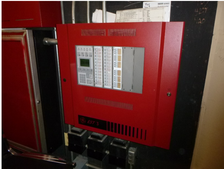
The EST fire alarm control panel.
