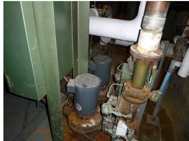
The original cold water booster pump skid package equipped with two pumps and controls.
