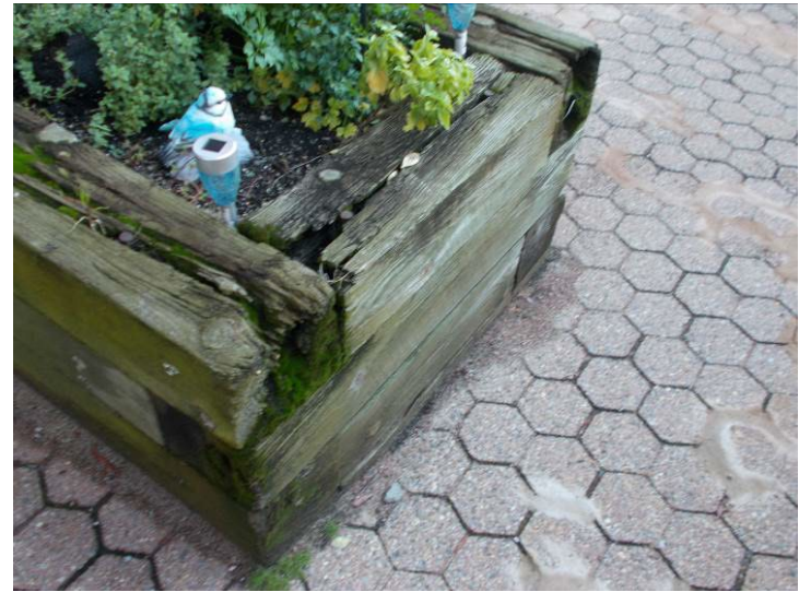
Flower box at the direct entry unit with wood tie retaining walls; note the deterioration.
