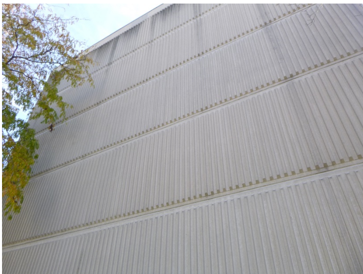
Typical condition of the precast concrete panels at an end wall. Note: Staining at upper section of the wall.
