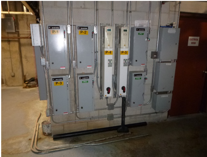
View of the variable frequency drives (VFDs) that govern two base-mounted 5-horsepower circulator pumps.
