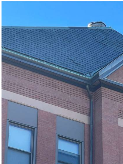
Lifting shingles at the front of the building will be repaired in 2022.
