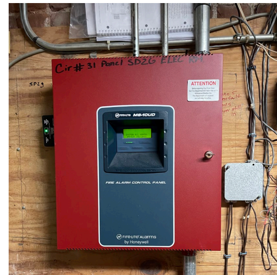
View of the FireLite MS-10UD fire alarm panel which was installed in 2015.
