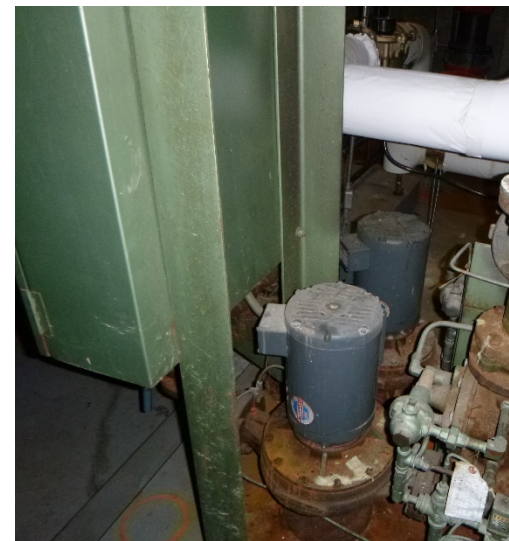
The original cold water booster pump skid with two pumps and control
