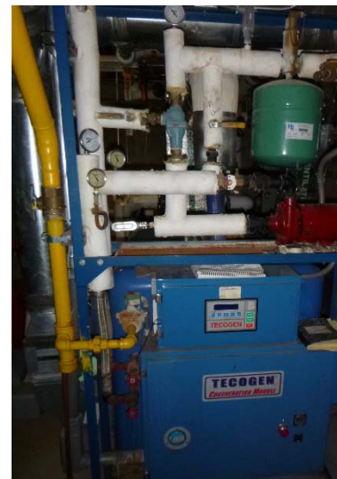
The Tecogen cogeneration system that produces domestic water and supplemental electricity for the building.
