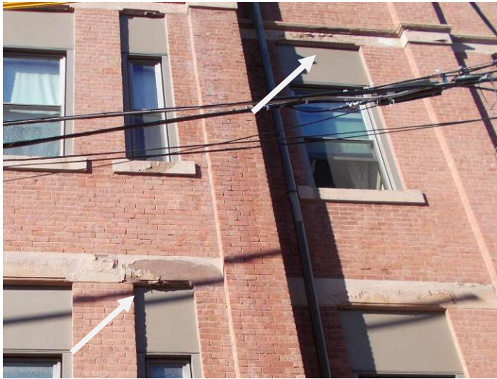
Areas of spalling and concrete damage at windows.
