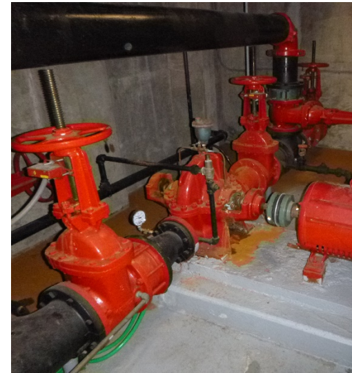
The original 50-horsepower split case
