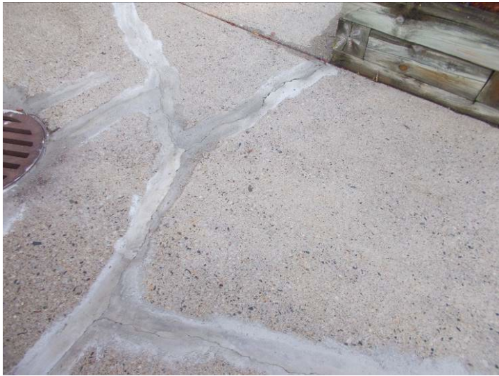
Pedestrian access provided by concrete walkways, previous cracking and repair efforts observed.
