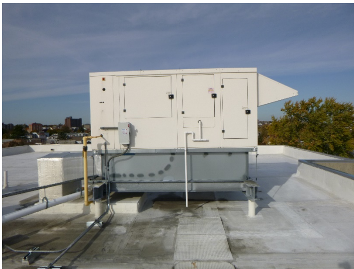
One of three recently replaced Reznor roof mounted makeup air units (MAUs).
