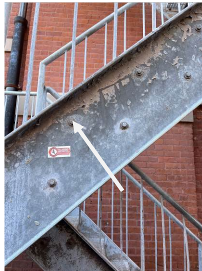
View of the aluminum fire escape at the rear of the building; note paint.
