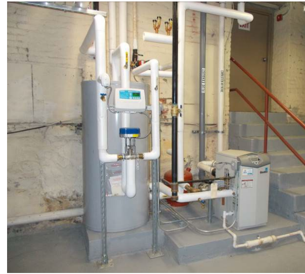
View of the Lochinvar domestic hot water boiler, storage tank, and Heat-Timer ETV Platinum Plus control valve.
