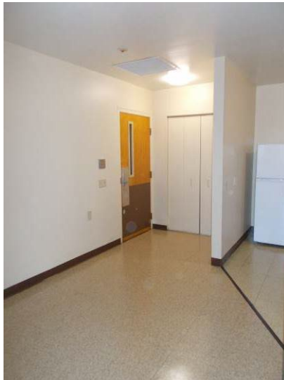
View of typical unit living area finishes. Note locking hardware on the entry door requires pinching and turning which is non-compliant.
