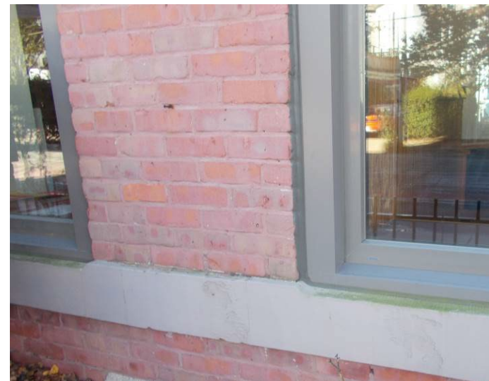
Vinyl framed windows are less than ten years old. The caulking appears to still be pliable.
