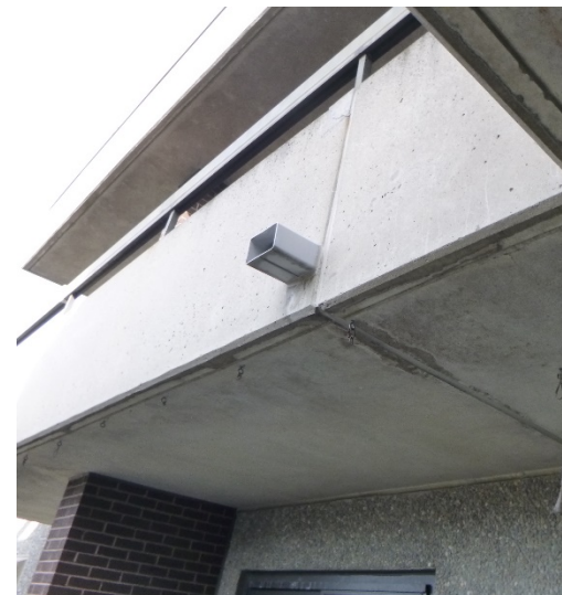
No significant cracking/deterioration was observed on the underside of balconies from available
