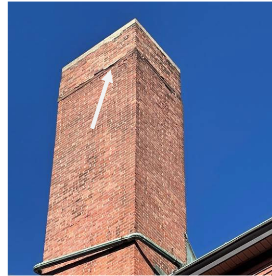
View of the chimney, note the mortar loss at the upper courses of brick.
