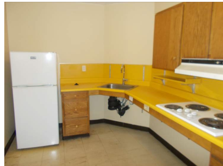
View of the community room kitchen.
