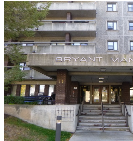
The front entrance. Note: the front entrance doors are scheduled to be refurbished in 2021. The concrete steps and landing are scheduled for replacement/rebuilding of the loading dock.
