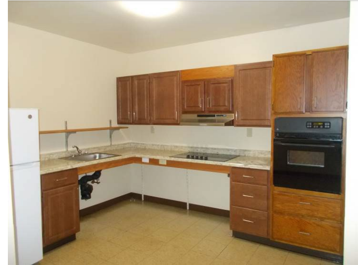
View of the accessible unit kitchen finishes and appliances.
