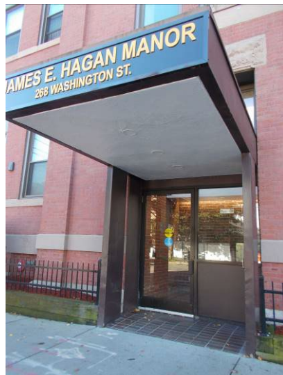
View of the entry canopy and main entry door.
