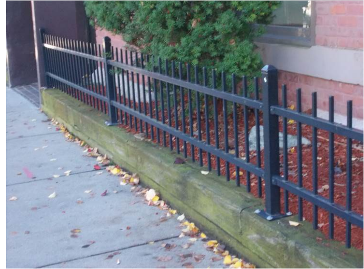
Newer aluminum fencing along the city sidewalk.
