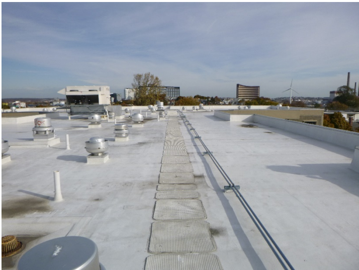
View of the upper roof surface.
