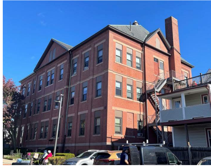
View of the West façade (side) and rear of the building.
