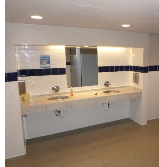
One of two recently renovated public restrooms.
