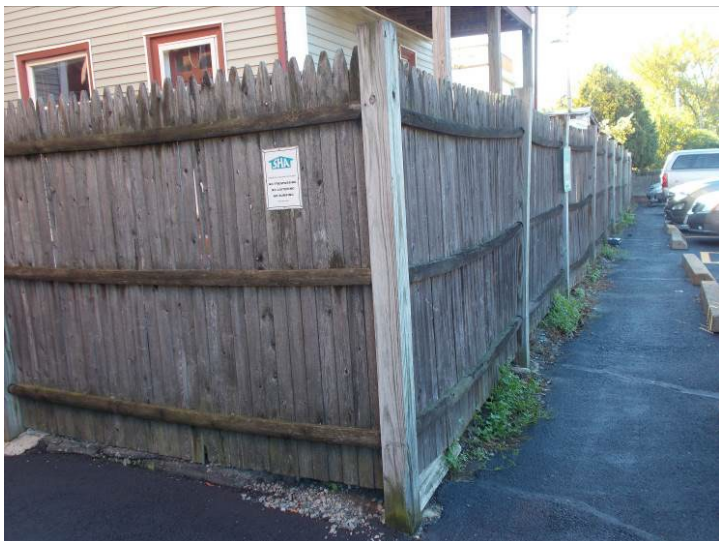
Wood stockade fencing along the parking lot and rear property lines.
