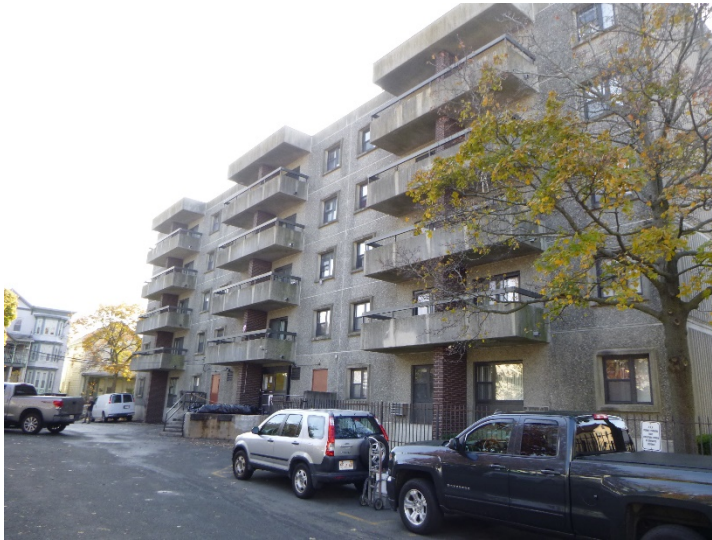
Typical building architecture as seen at the north elevation.
