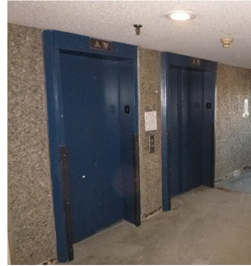
The fourth-floor elevator lobby and hallway replaced at the time of the renovation.
