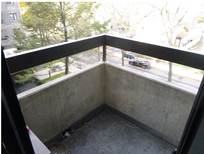
View of a concrete balcony and metal railing system.
