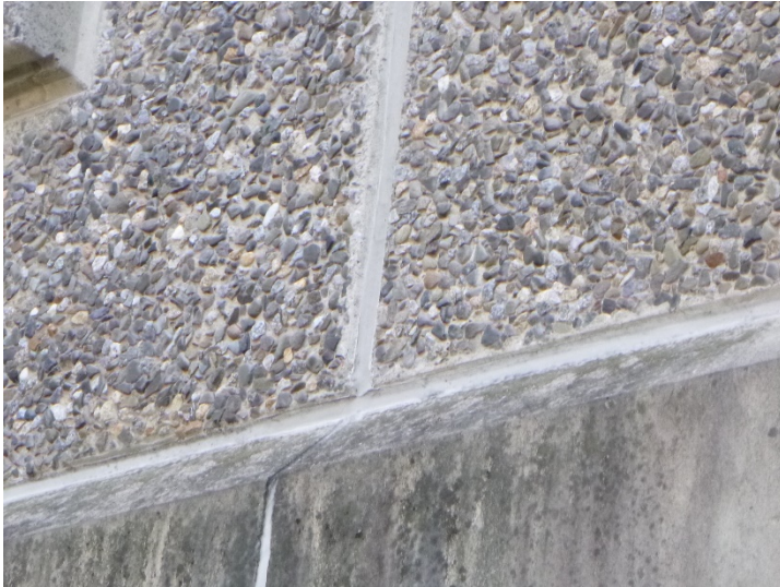
Close up of the caulking joints between precast panels.
