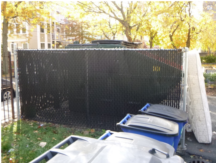
View of the dumpster enclosure.
