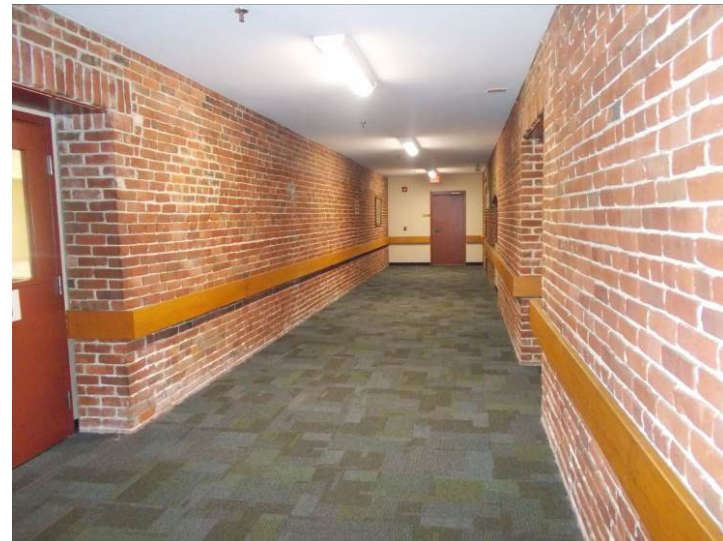
View of typical common hallway finishes.
