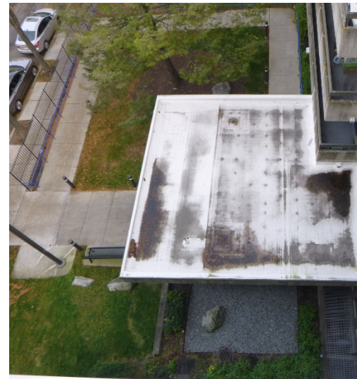
View of the entrance canopy roof
