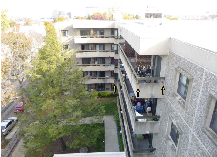
View of the concrete balconies. Concrete surfaces exhibit staining and organic growth. Yellow arrows indicate rust staining near balcony railing mounting brackets.
