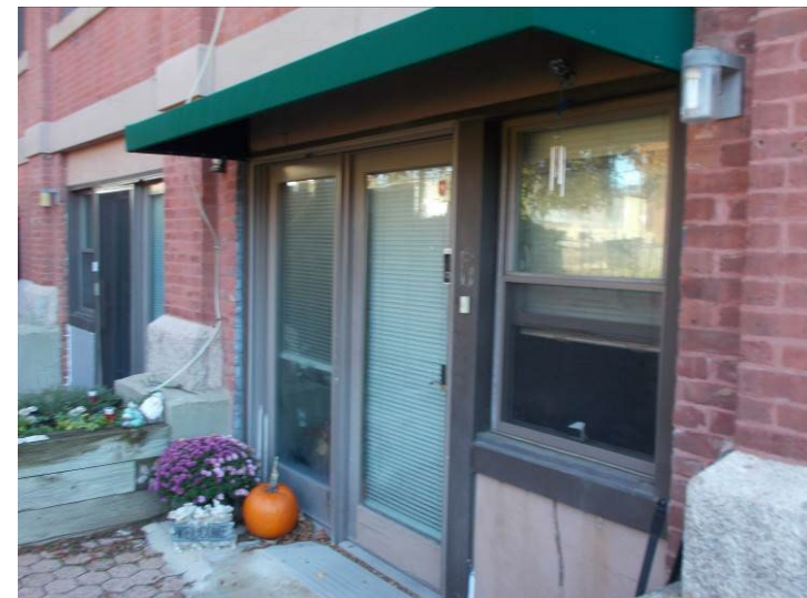
View of the lower-level unit entry doors; note one unit protected by a canvas awning.
