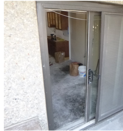
Typical sliding glass dwelling unit balcony
