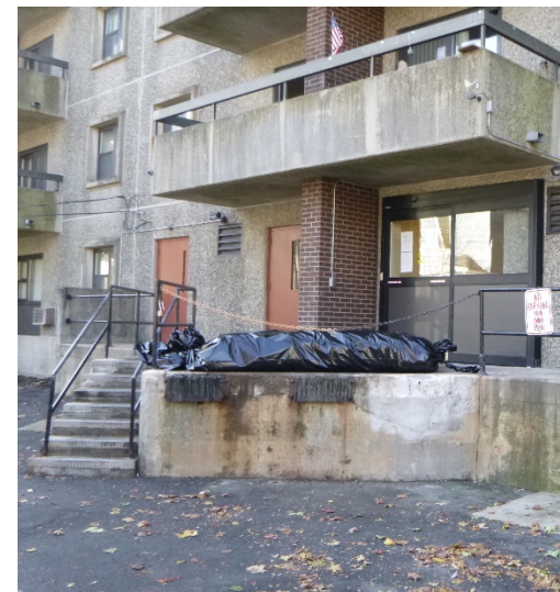
View of the side entrance and loading dock. The concrete steps and landing are scheduled to be rebuilt.
