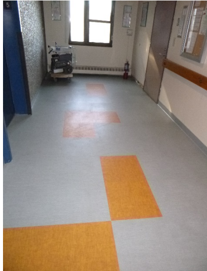
View of the fifth-floor elevator lobby with recently installed linoleum tile flooring.
