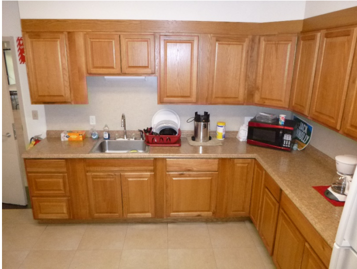
The community room kitchen cabinetry.
