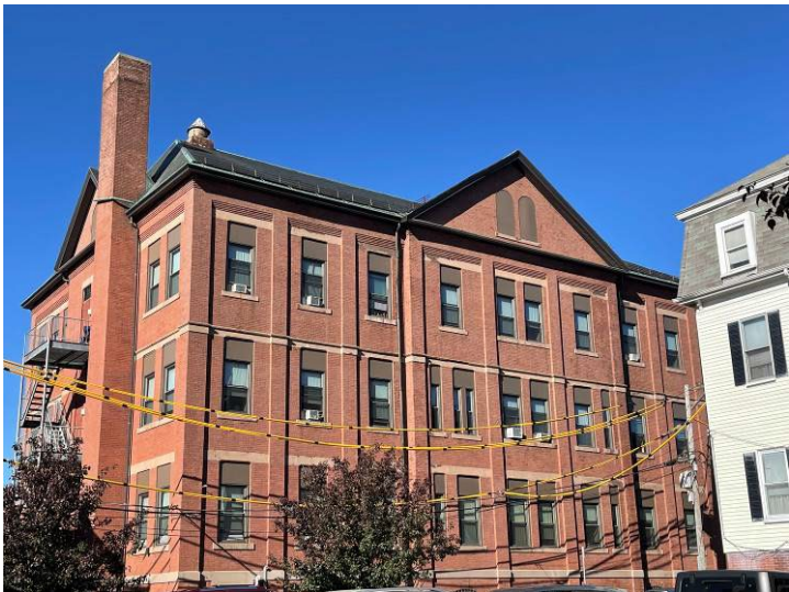
View of the Kingman Road facade
