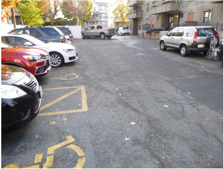
View of the asphalt paved north parking lot.
