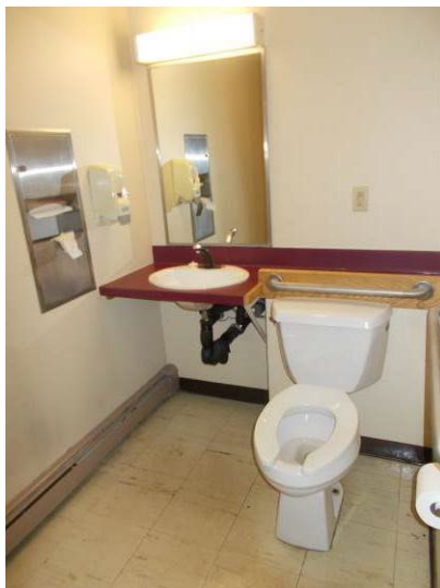
View of one of two common restroom finishes and fixtures.
